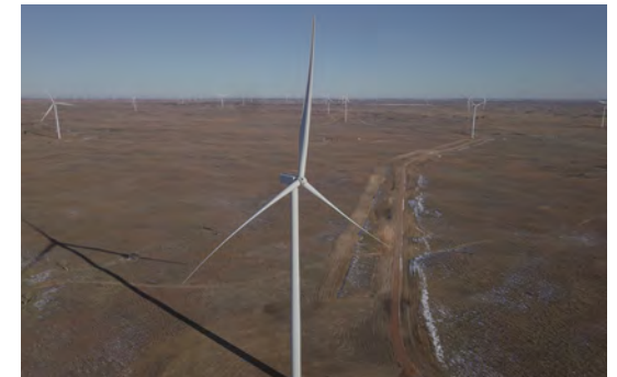
Boiling Springs Wind Farm (120 MW)
