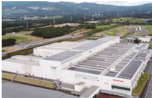
Kumamoto Factory (5.35 MW)
